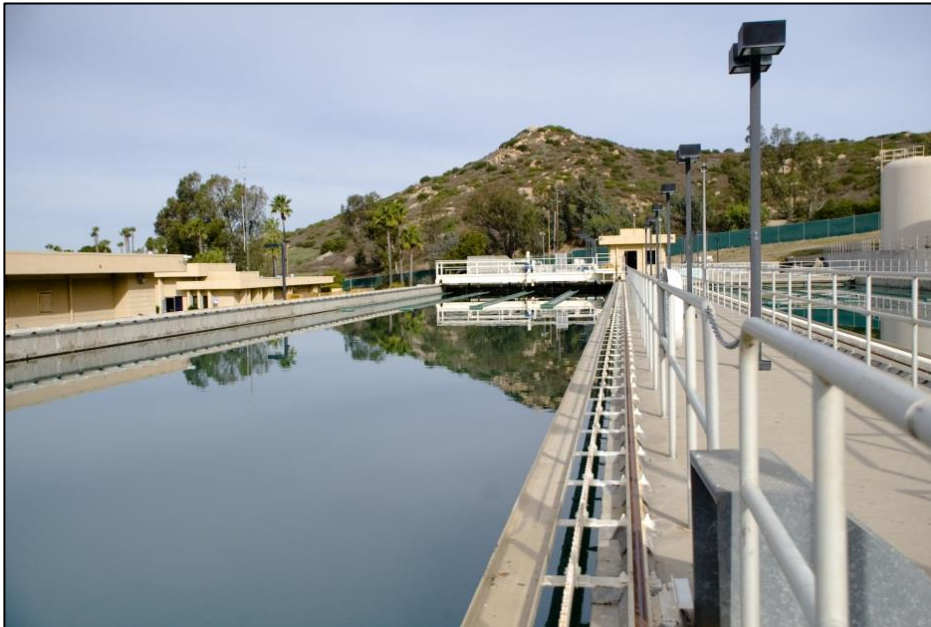
The City's Lester J. Berglund WTP is located at Lake Poway, which stores raw water purchased from SDCWA.
