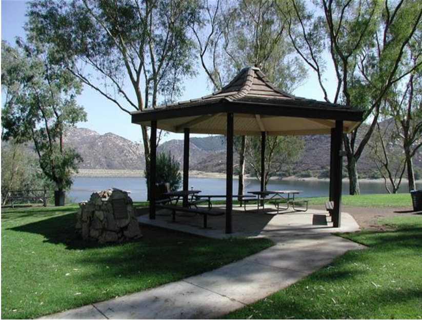
Lake Poway, utilized for raw water storage, has adequate emergency water supplies for the City for up to six months.
