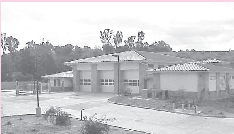
Fire Station No. 3, dedicated in 2004, is a highlight of Poway's commitment to public safety.
